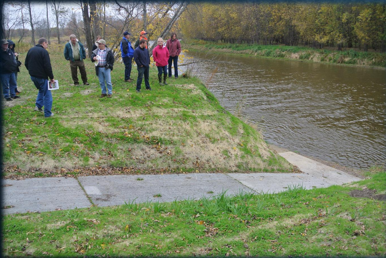
New Canoe Access, replaced washed out access
