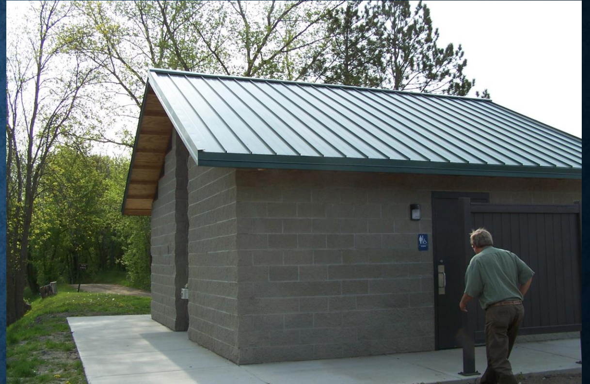
New showerhouse/restroom facility Aitkin County Campground
